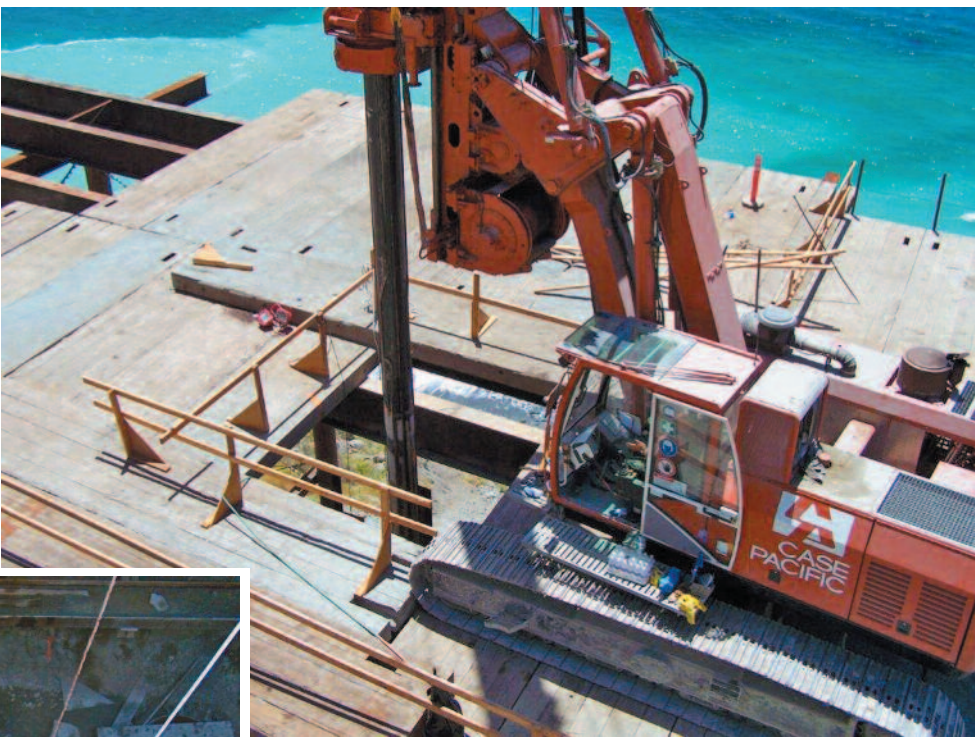
Bauer BG 20 on trestle working platform Bent 3.
