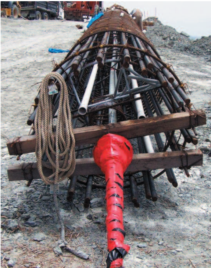
Rebar cage for the Bent piles at Pitkins Curve Bridge showing the congestion and tiedown anchor.
